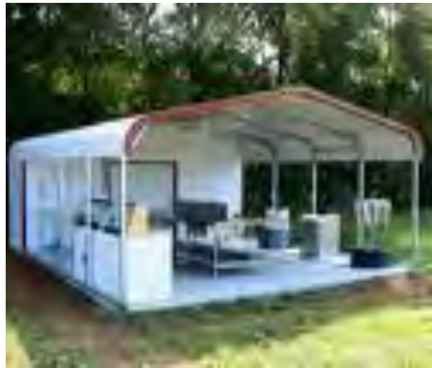
Shed on Concrete Pad
